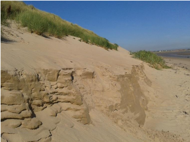
Plate 8 – Survey photograph 1aBTBC38_20150930_N3
